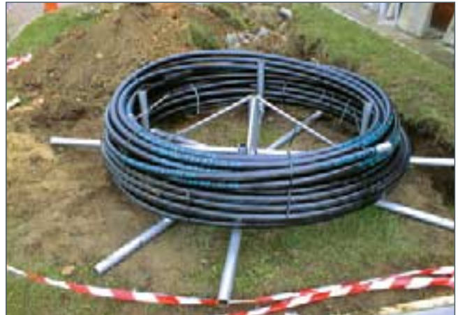
Fig.2: A simple jig facilitates uncoiling of the flexible LPG piping on site.
